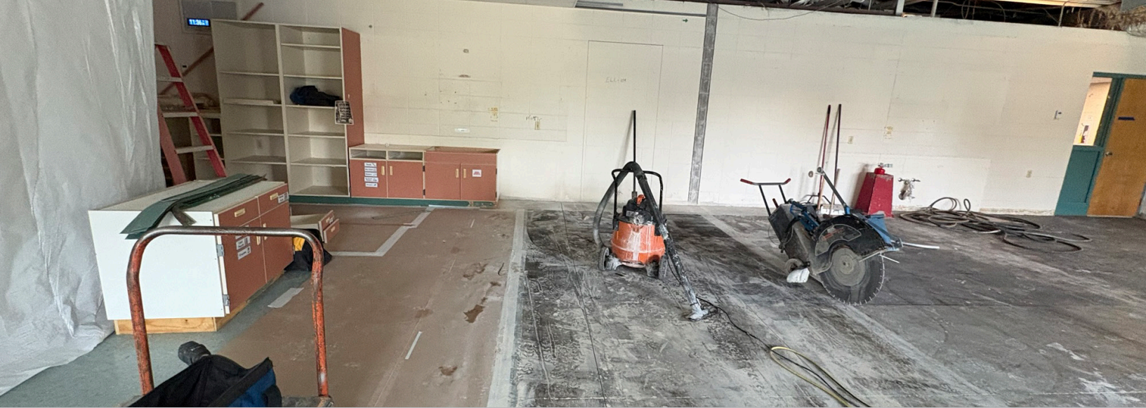
EARLY LEARNING CENTER DEMOLITION
