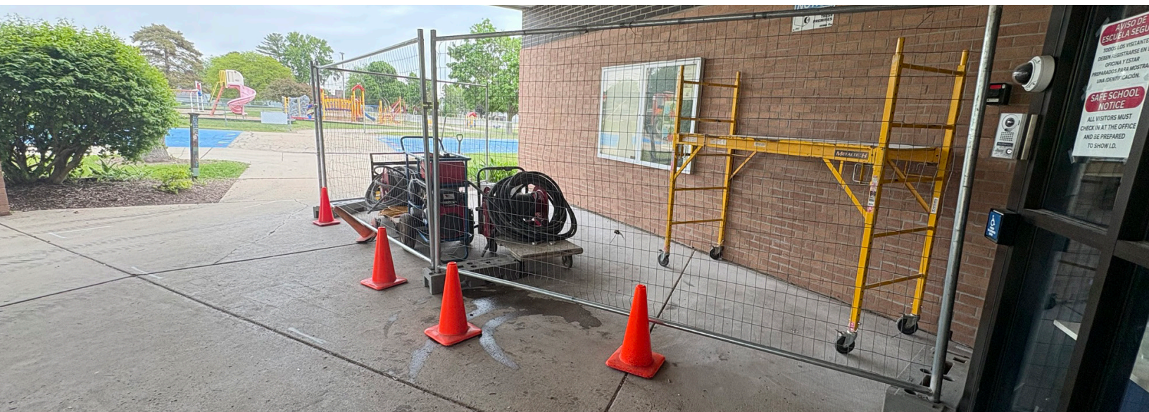
EARLY LEARNING CENTER EXTERIOR DEMOLITION
