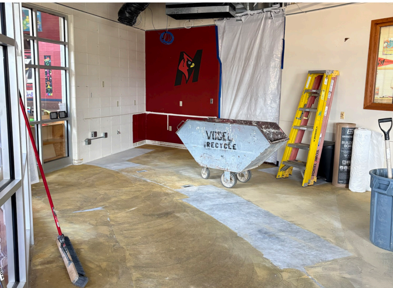
ELEMENTARY SCHOOL DEMOLITION
