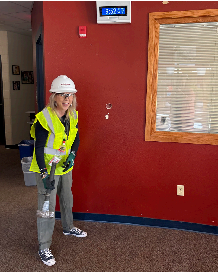
MRS. NEEDLES KICKS OFF DEMOLITION
