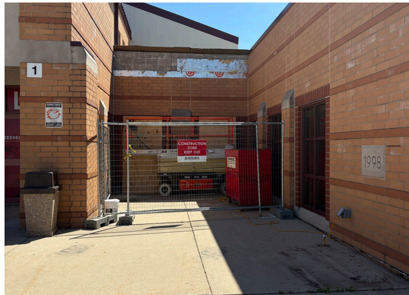
HIGH SCHOOL DEMOLITION
